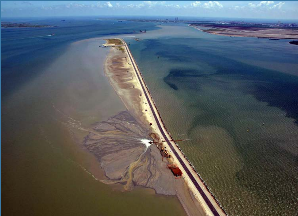
Texas City Dike
