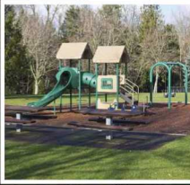
Example Playground Equipment
