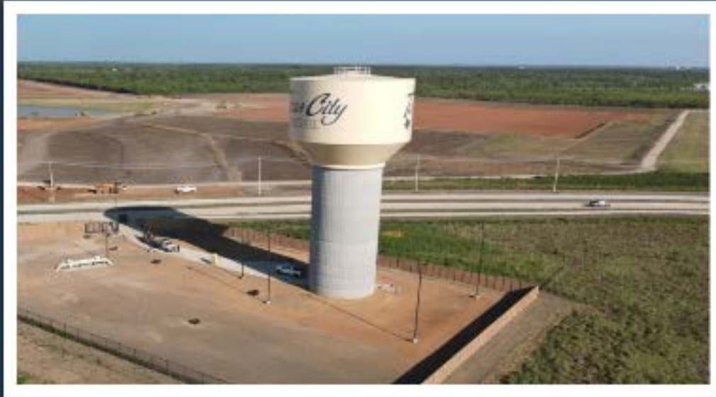
Lago Mar Elevated Tank (2021-2022)
