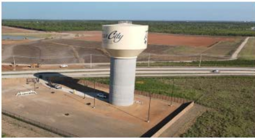
Lago Mar Elevated Tank (2021-2022)
