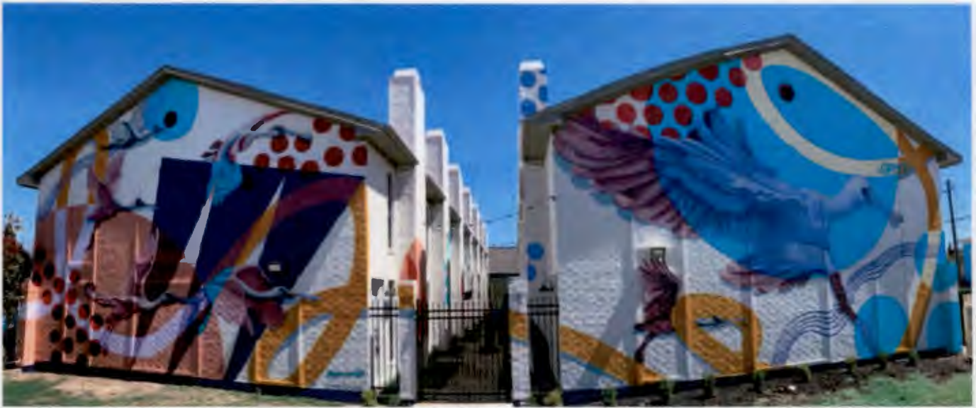
"To the Beach" aerosol/latex on exterior 50' X 45' !0th and sealy Galveston ,Texas
