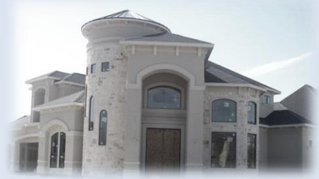
JC LATH & PLASTER.
