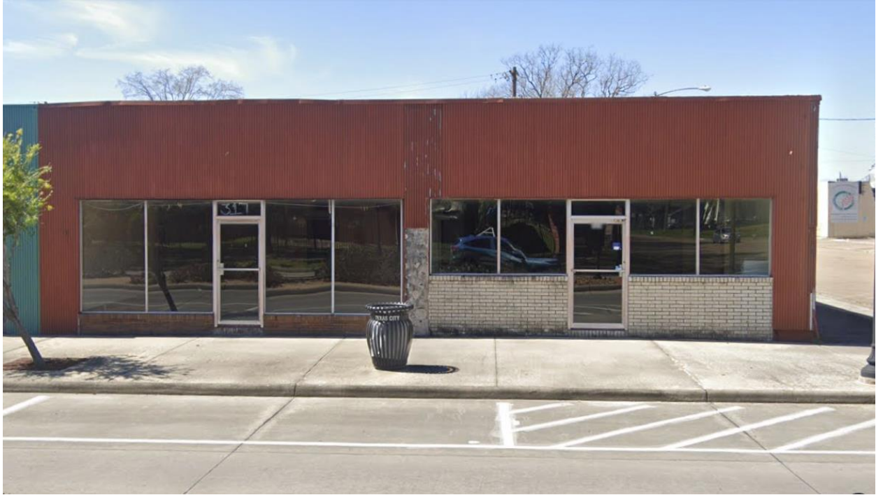
317 6 th Street (left) and 319 6 th Street (right). Properties are immediately adjacent, connected internally and share a storage area on the back half.
