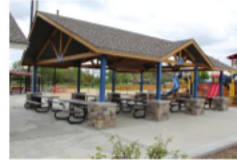
Open timber truss with column
