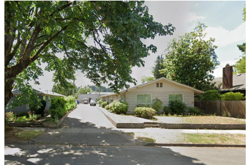
A MUR property on C Street
