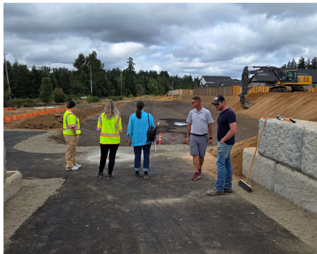
Construction Site Runoff Control
