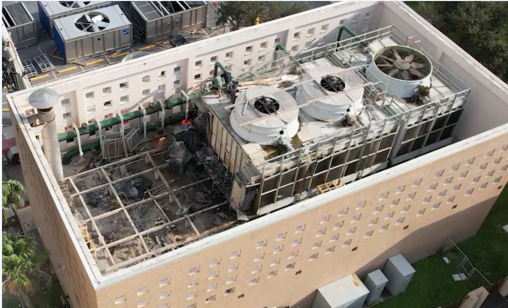
* Old Cooling Towers 1 and 2 removed.
