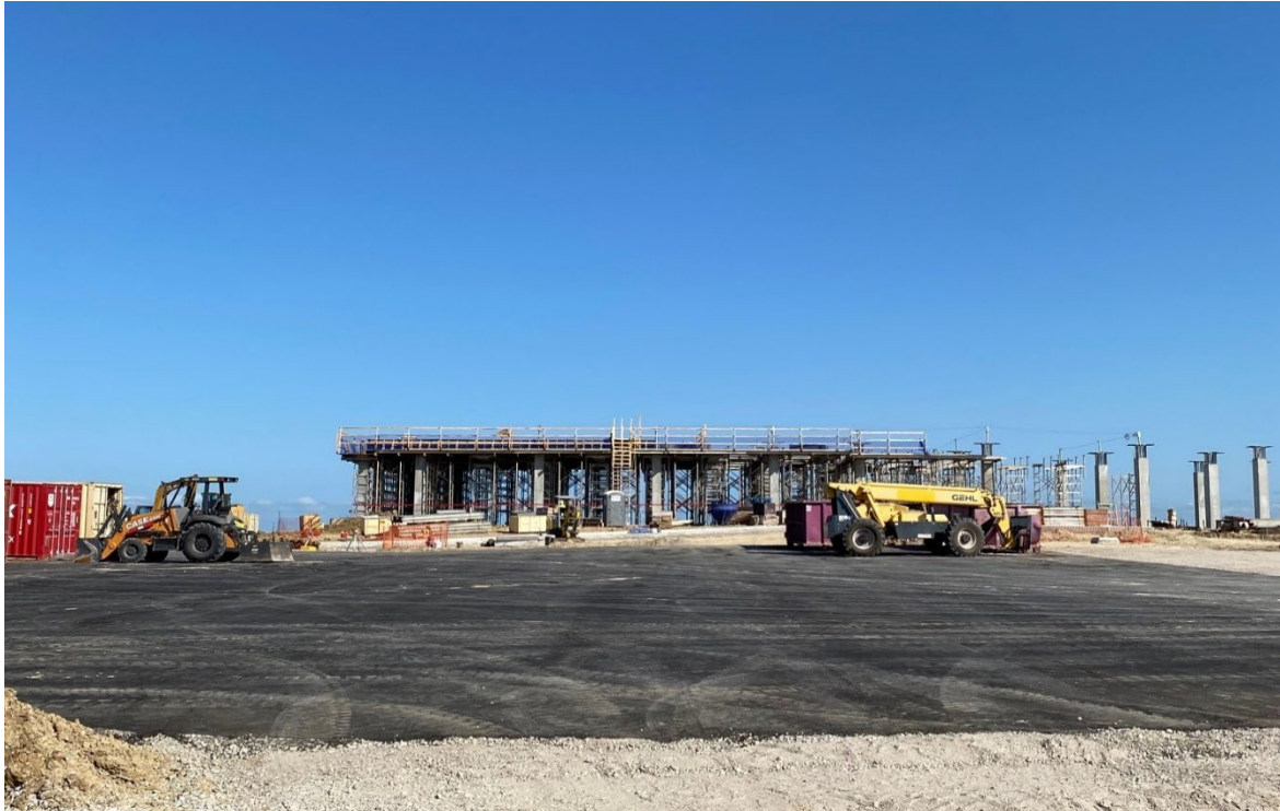
Plan west first asphalt lift Installed for laydown; level 2 podium formed
