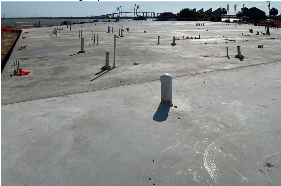
Convention center slab on grade poured
