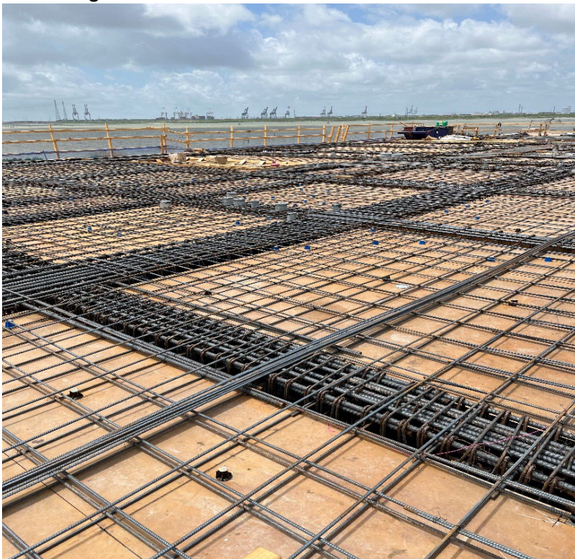
Reinforcing install on level 2 deck
