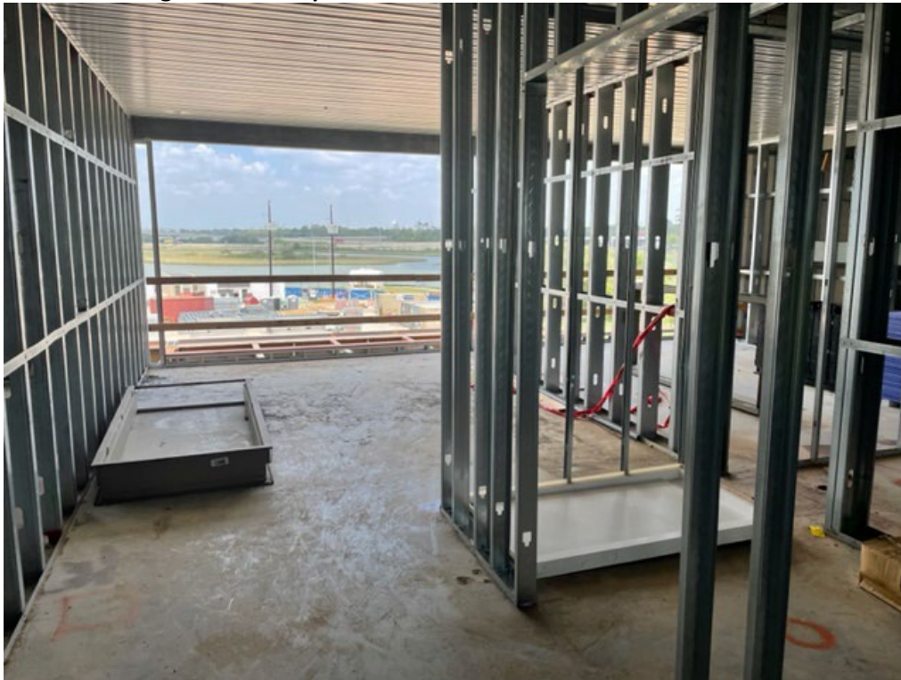
Level 2 Framing and shower pans installed
