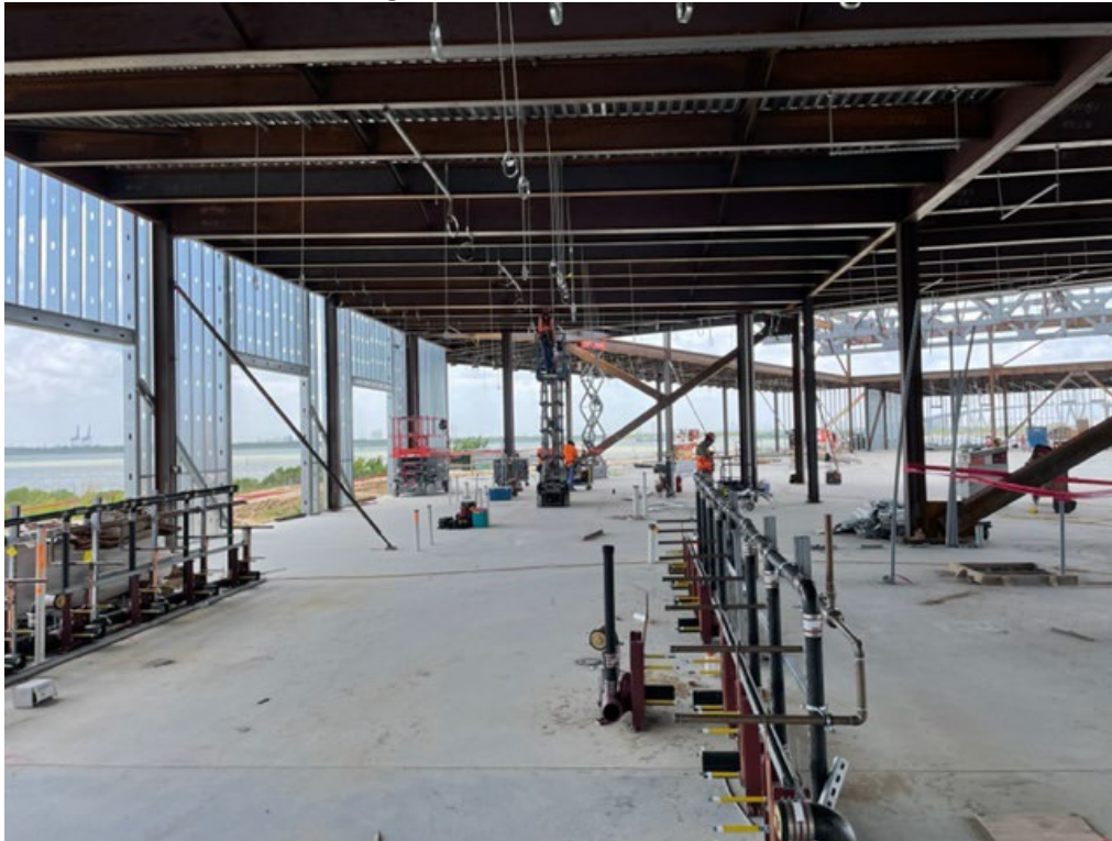
Convention Center MEP Hangers Installed
