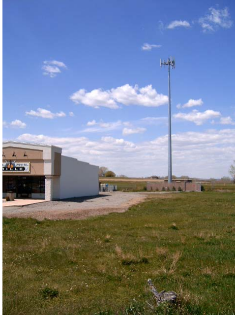
View west of cell tower at north end of subject property
