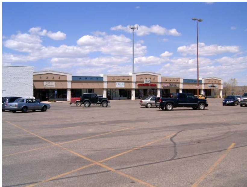
View northeast at existing strip retail center
