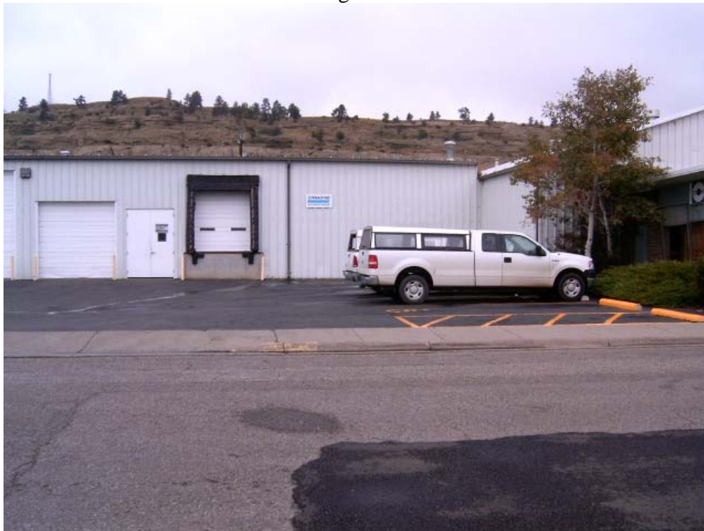
View north across 2 nd Avenue North
