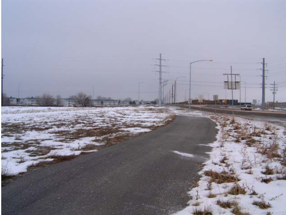
View east along multi-use trail on King Avenue West
