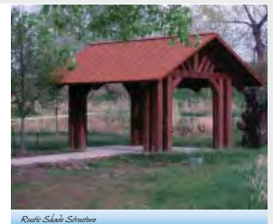
Rustic Shade Structure
