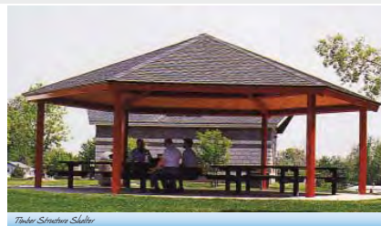
Tinder Structure Shelter
