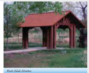
Rustic Shade Structure
