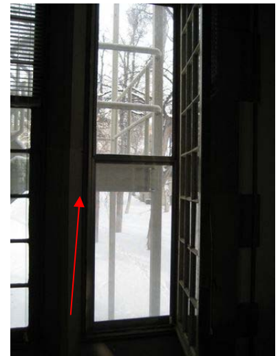
Casement windows to be weather-stripped
