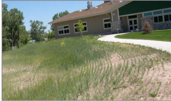
Drill seeding is the preferred method of native grass establishment
