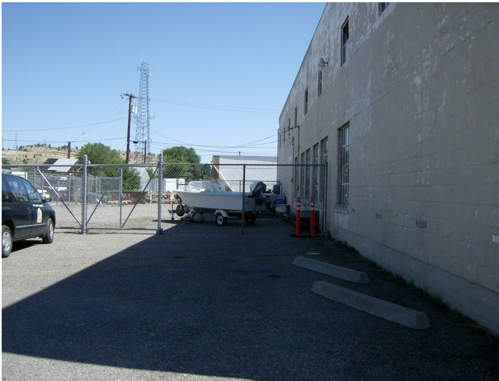
View of north side of existing building
