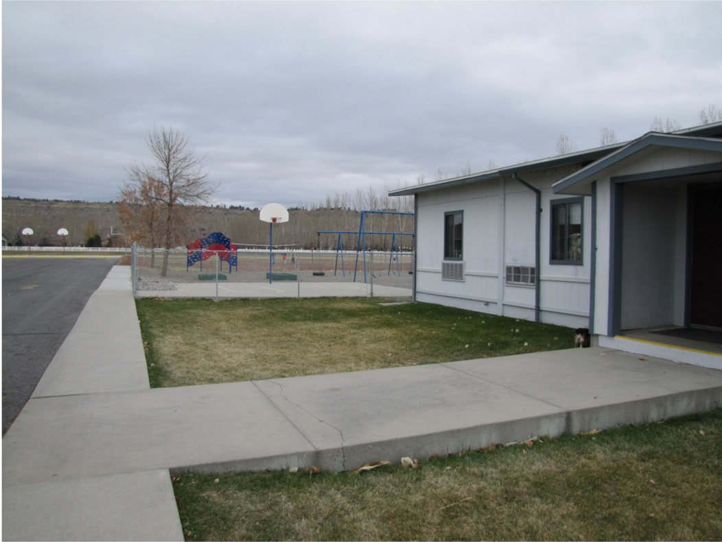
View north from building entrance
