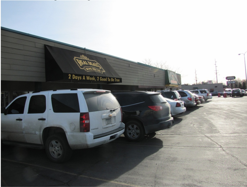
View south and east along existing building
