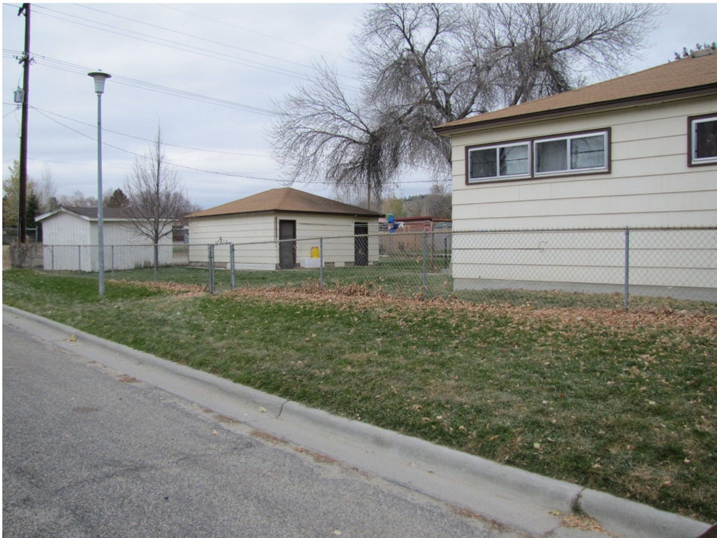
View of west (rear) of property at 2302 Meadowood
