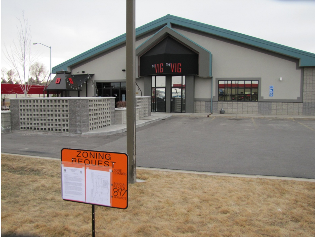
View of subject property – west from access drive
