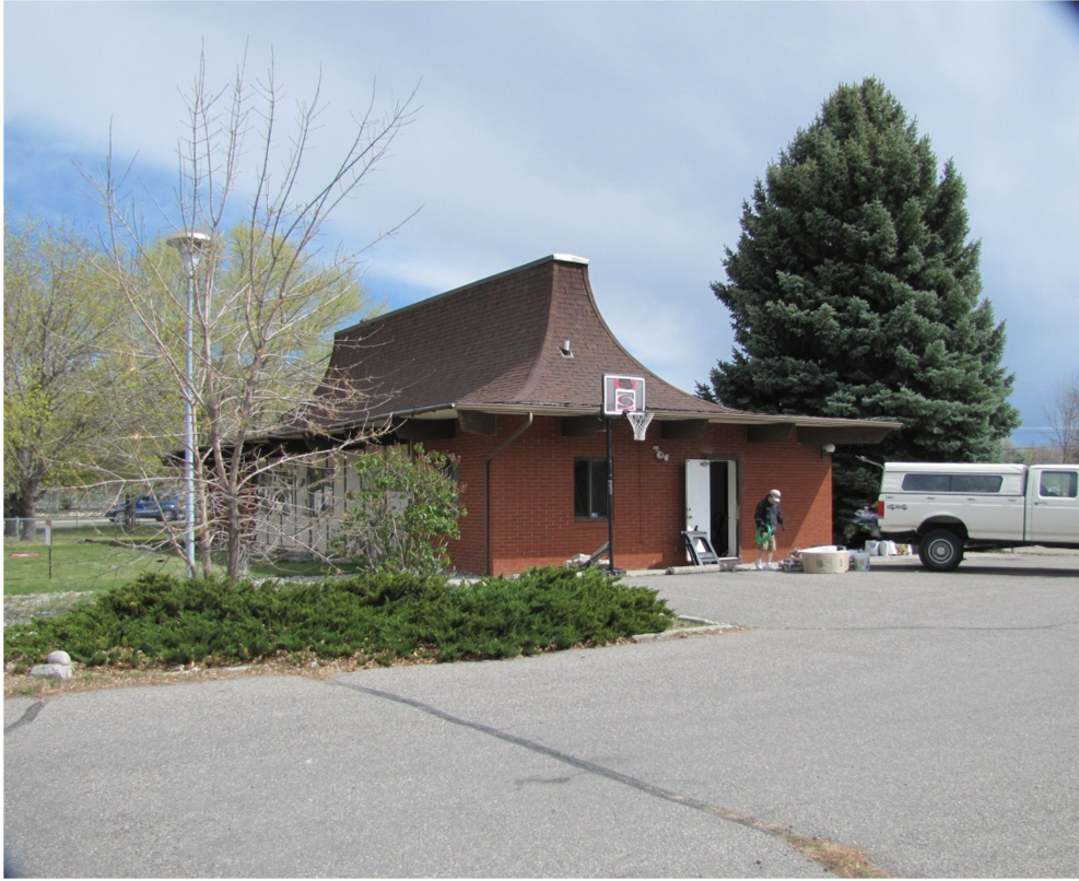
View from parking area west of building
