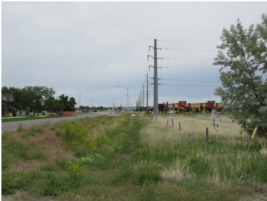
View east along King Avenue West
