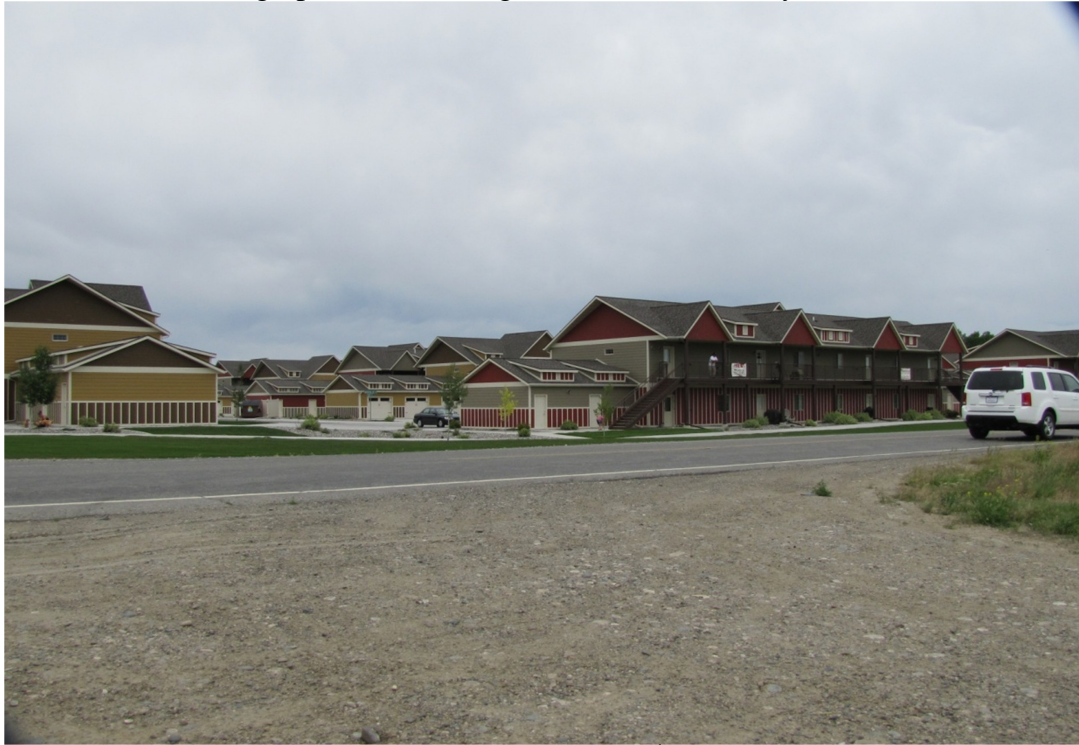
View north and east from S 44 th Street West
