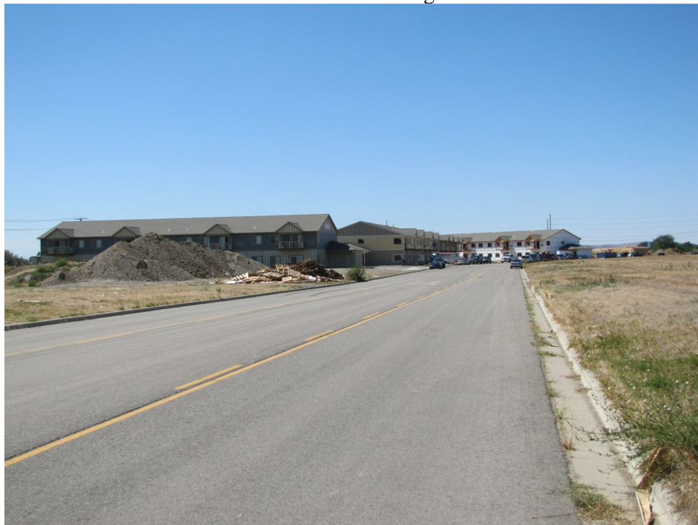
View west to multi-family apartments under construction
