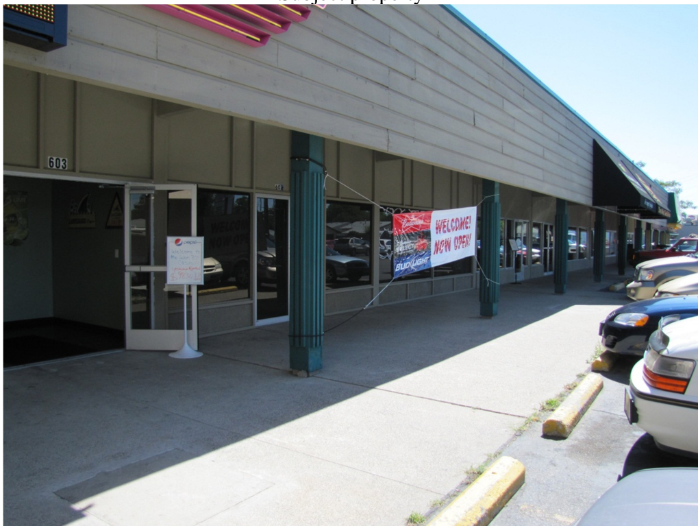
View south along front of building
