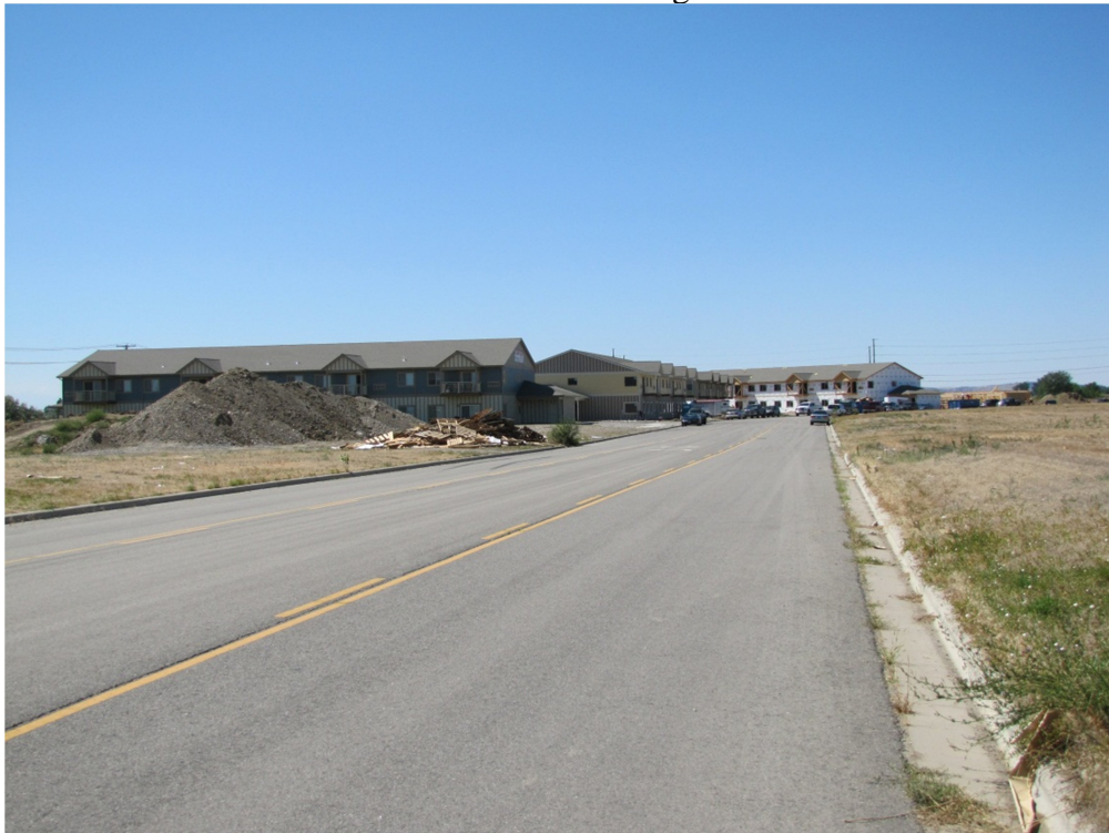
View west to multi-family apartments under construction
