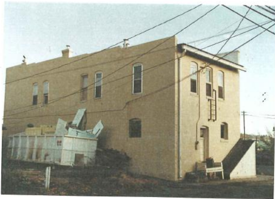
Viewing the south and west elevations from the alley.
