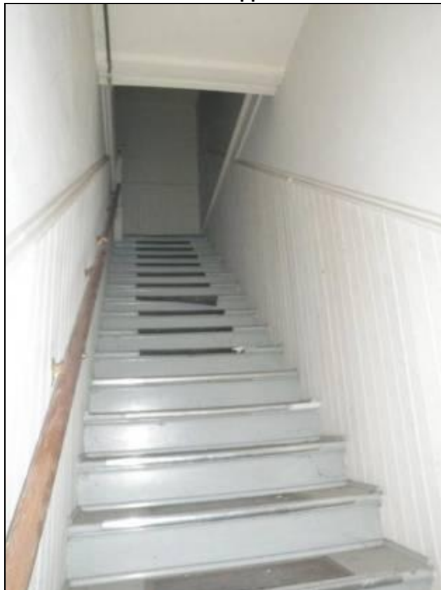
Stairwell to Upper Floor
