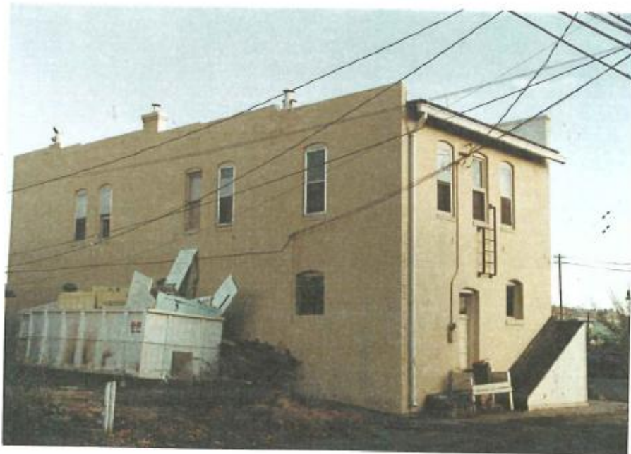
Viewing the south and west elevations from the alley.
