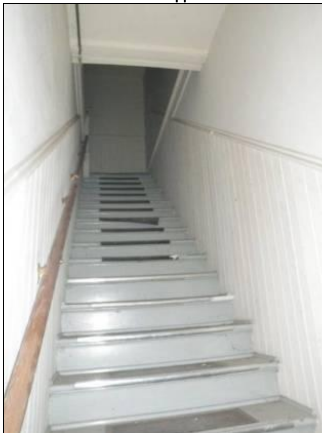
Stairwell to Upper Floor
