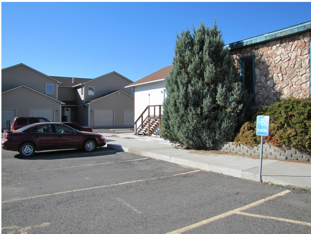
View of south west corner of vacant church/daycare building
