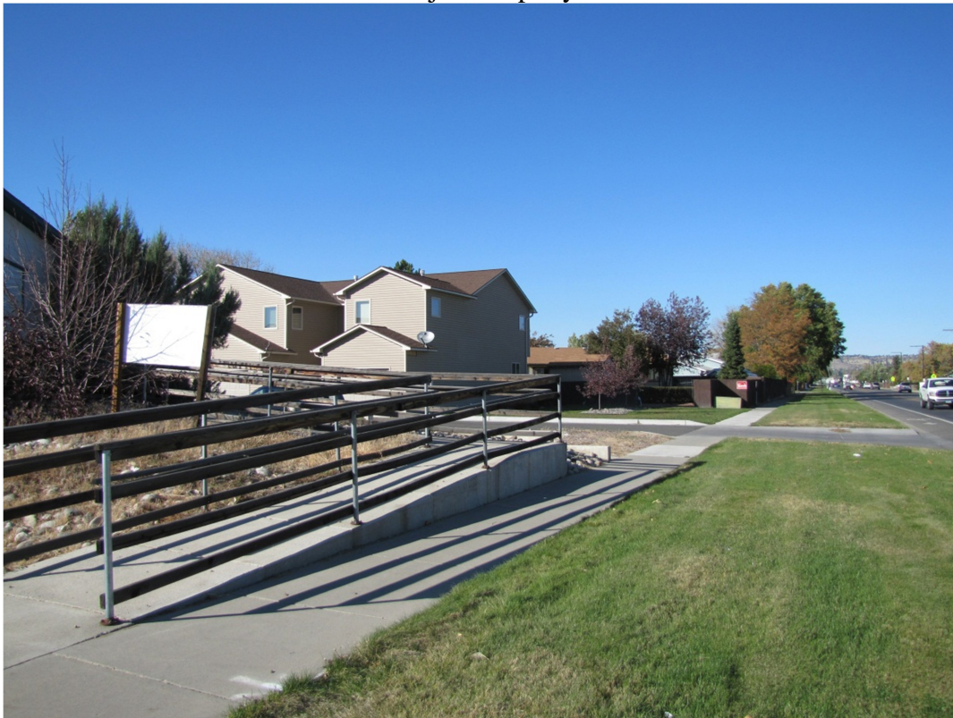
View north along 32 nd Street West
