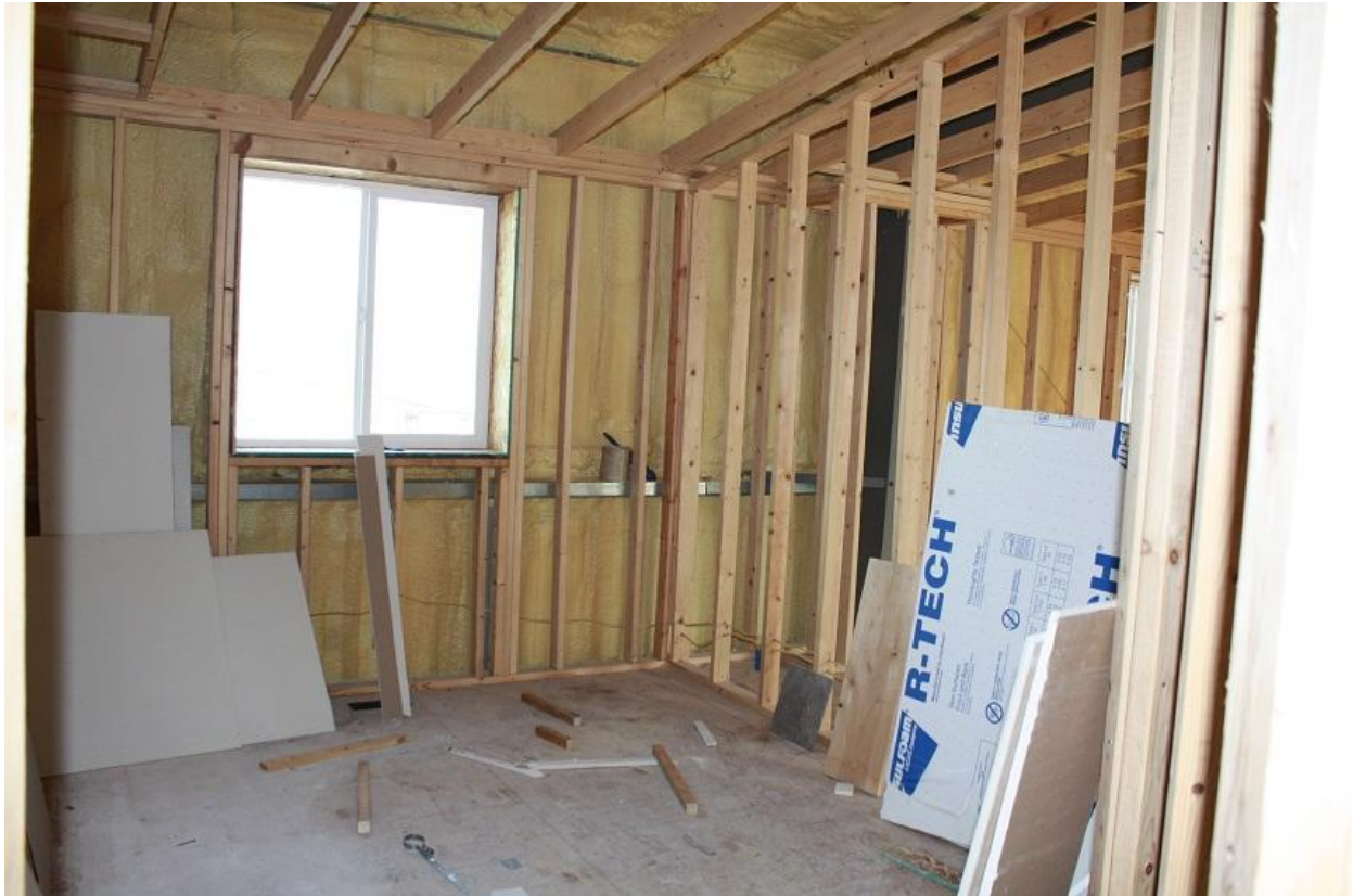
Garage Interior – Upper Level
