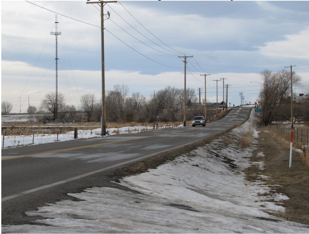
View west along Hesper Road to intersection with Shiloh Road
