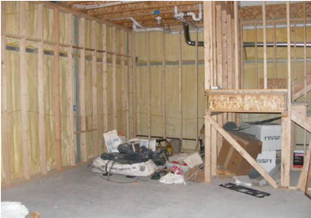
Garage Interior – Lower Level – Hobby Area
