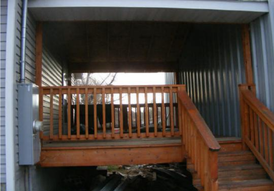
Covered Deck / Breezeway
