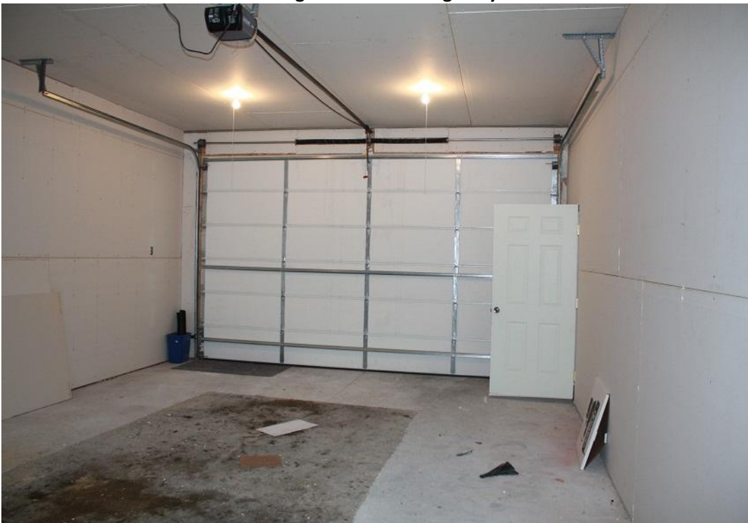
Garage Interior – Garage Bay
