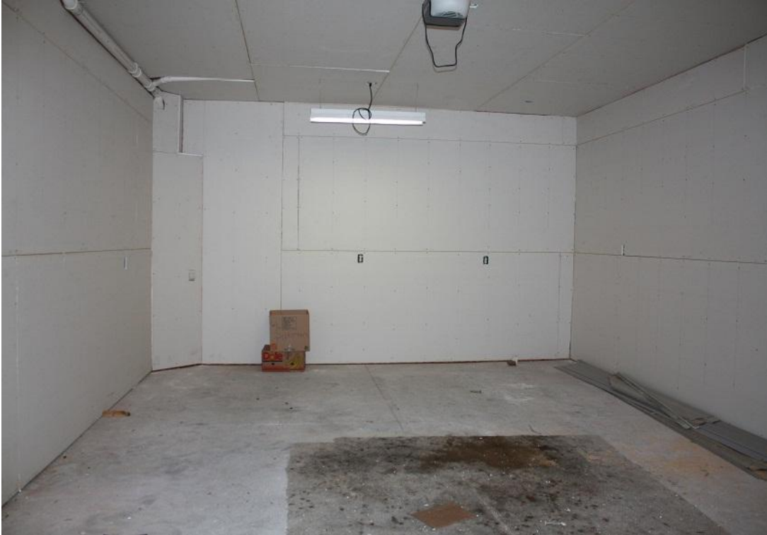
Garage Interior – Garage Bay
