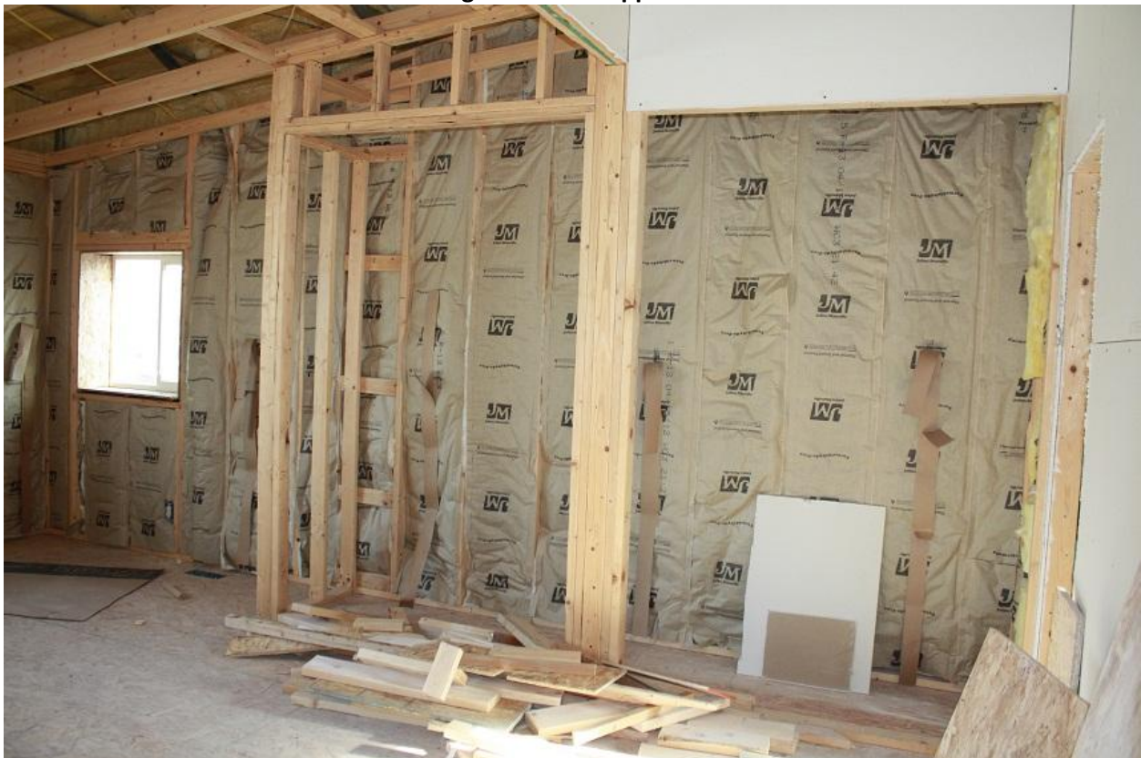
Garage Interior – Upper Level
