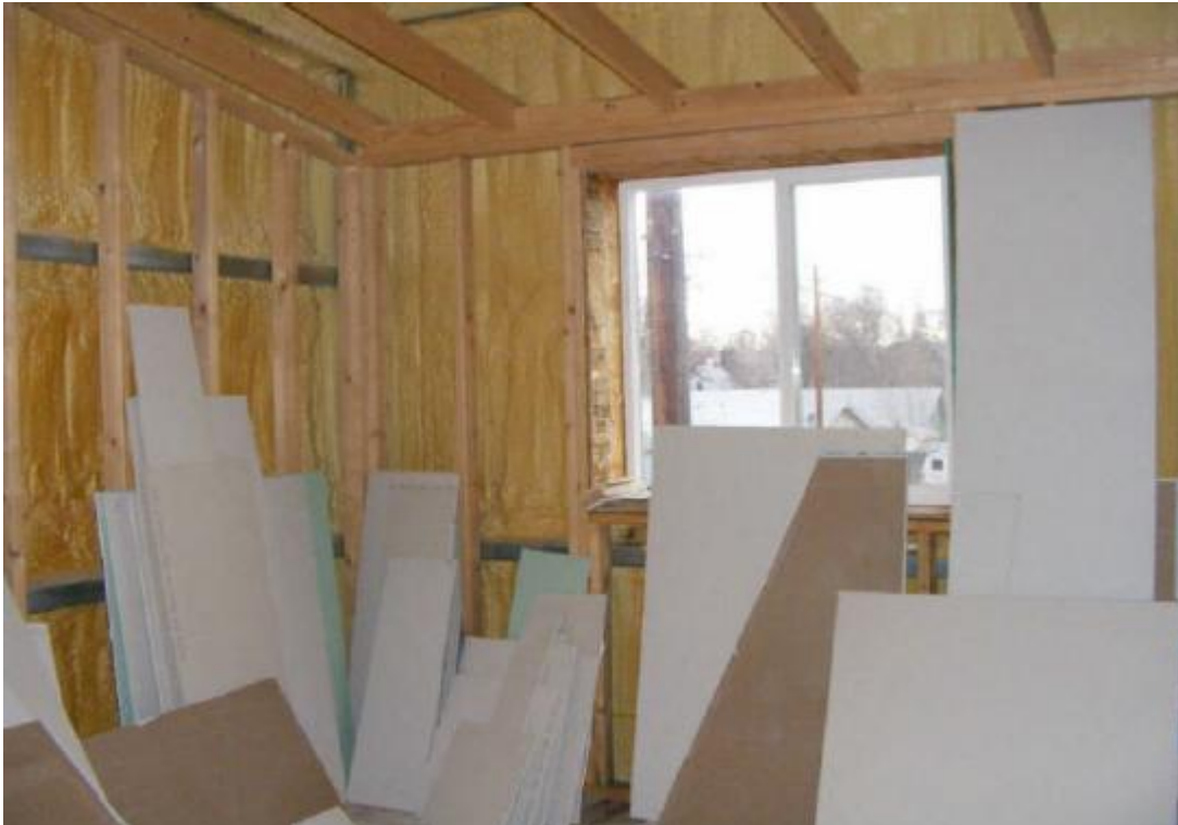
Garage Interior – Upper Level
