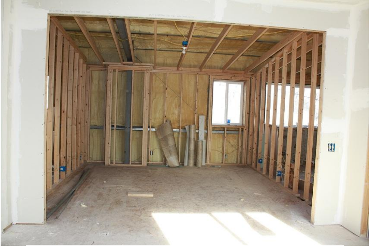
Garage Interior – Upper Level
