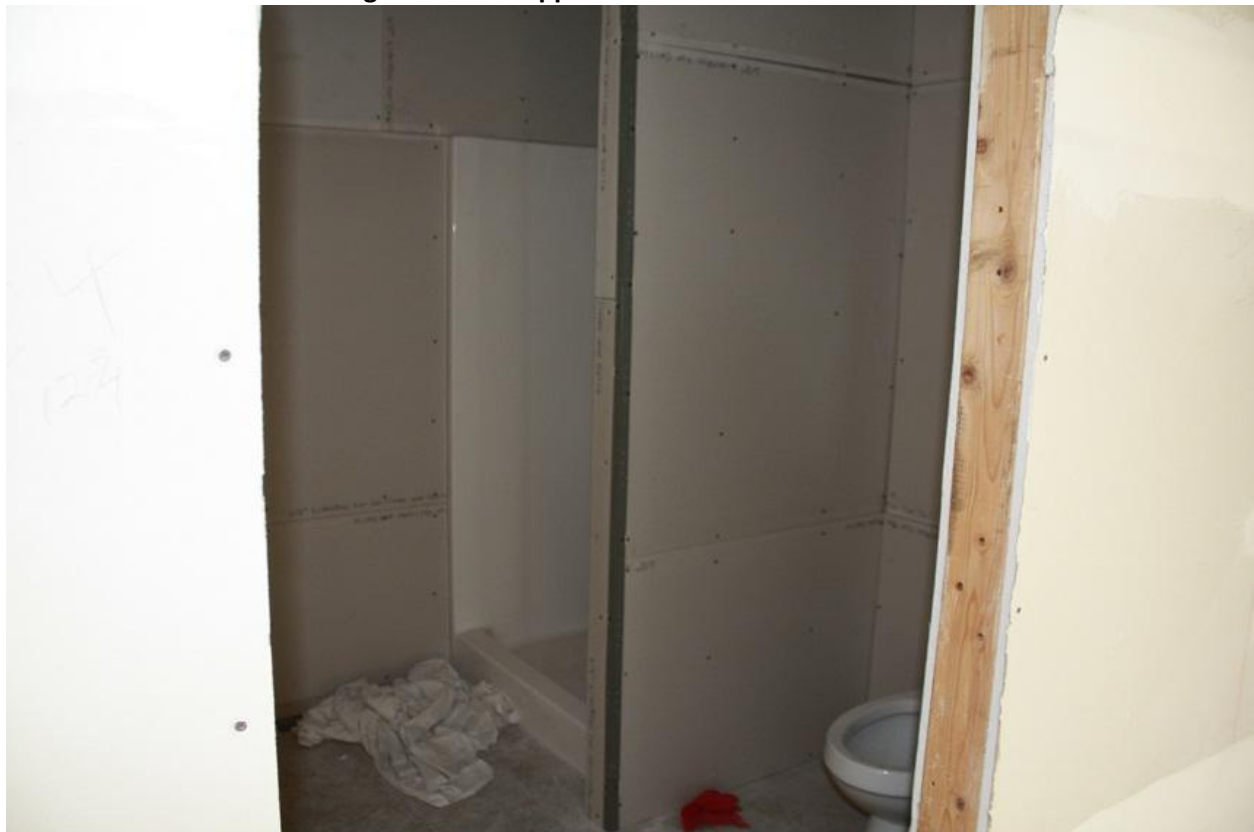
Garage Interior – Upper Level – Unfinished Bathroom
