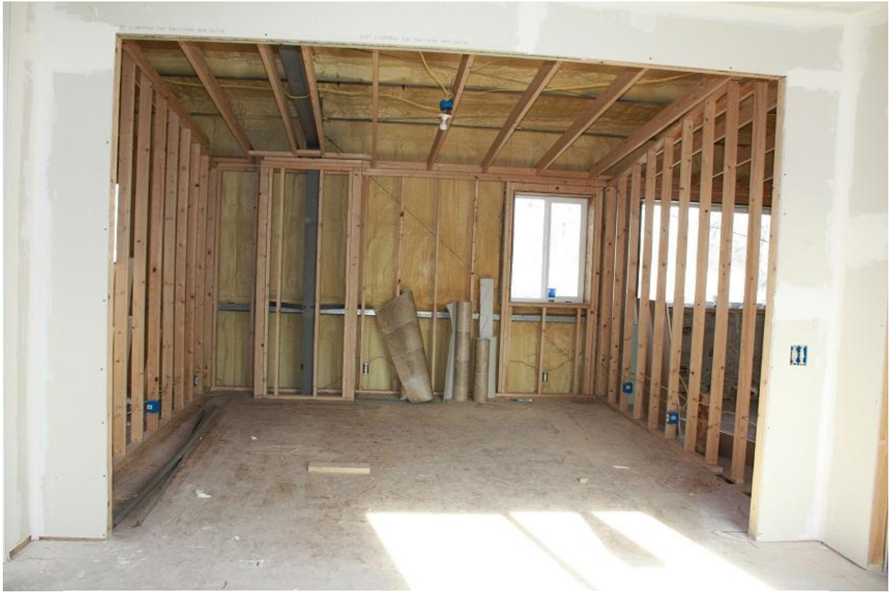
Garage Interior – Upper Level
