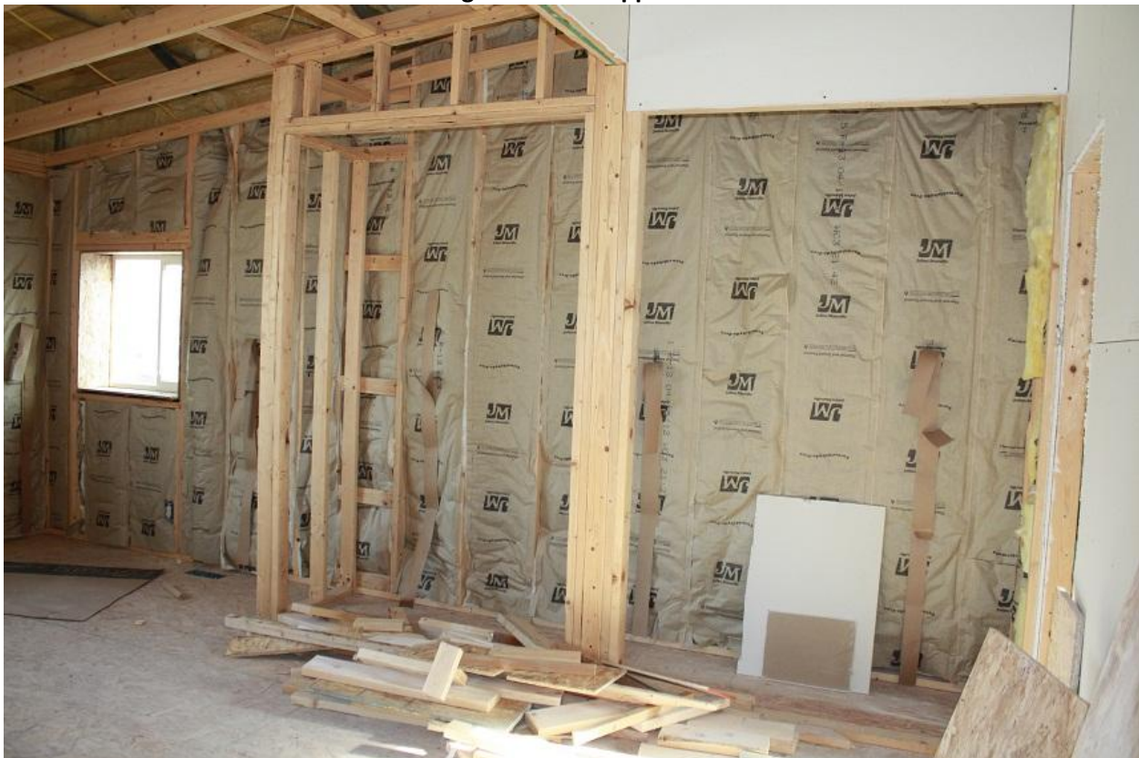
Garage Interior – Upper Level
