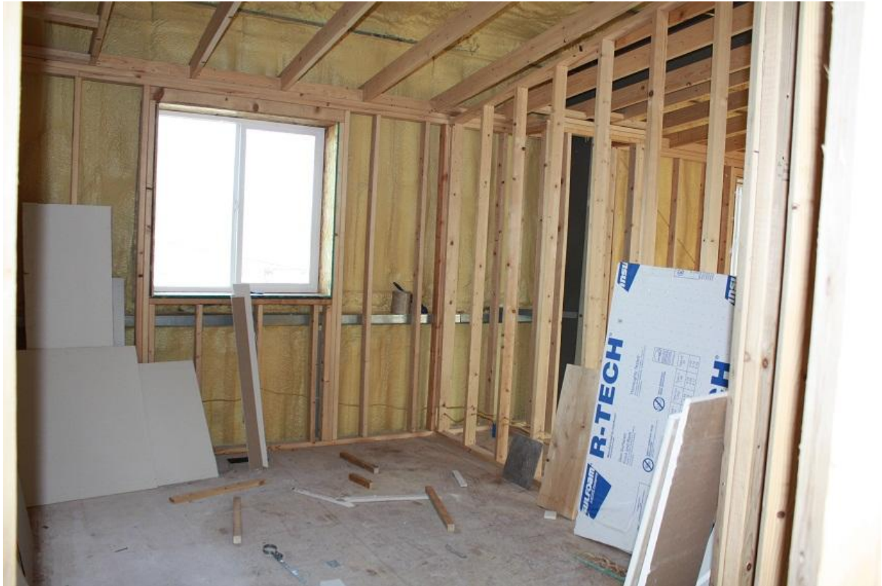
Garage Interior – Upper Level
