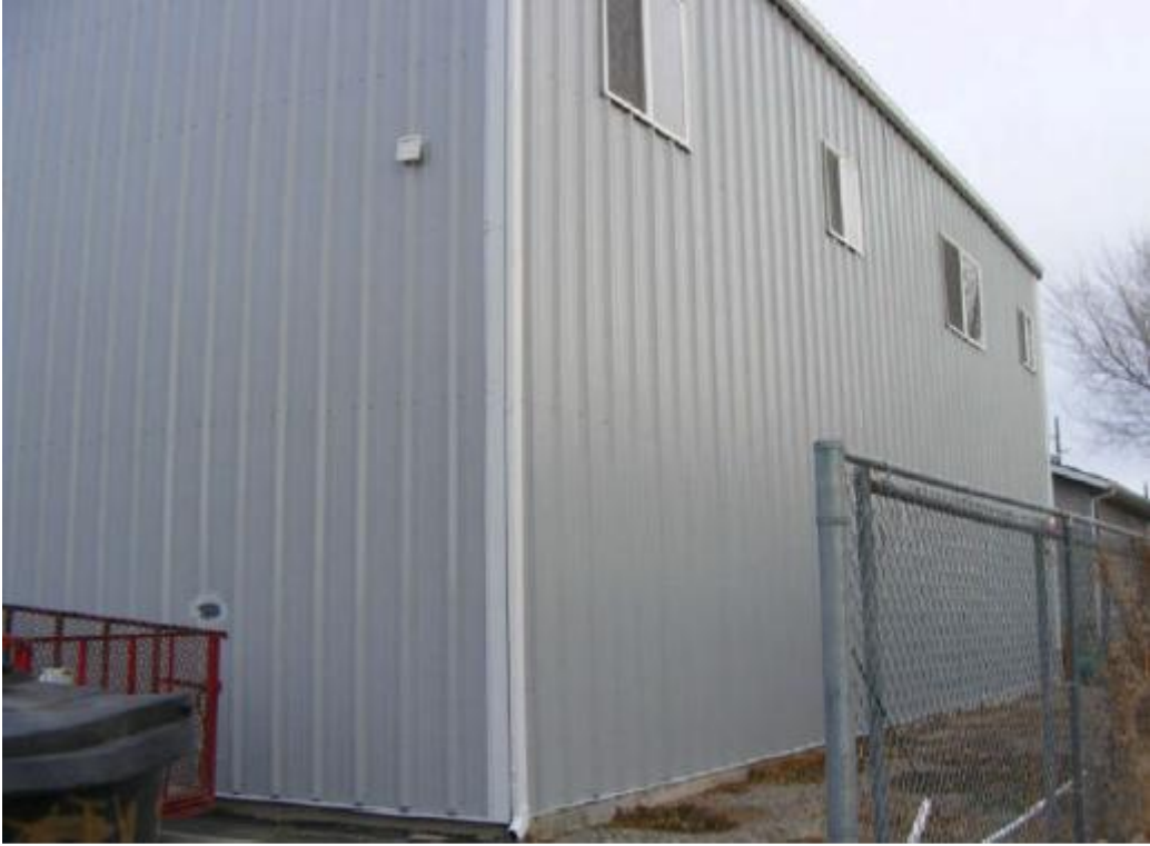
Garage Exterior - Rear
