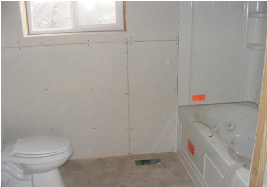
Garage Interior – Upper Level – Unfinished Bathroom
