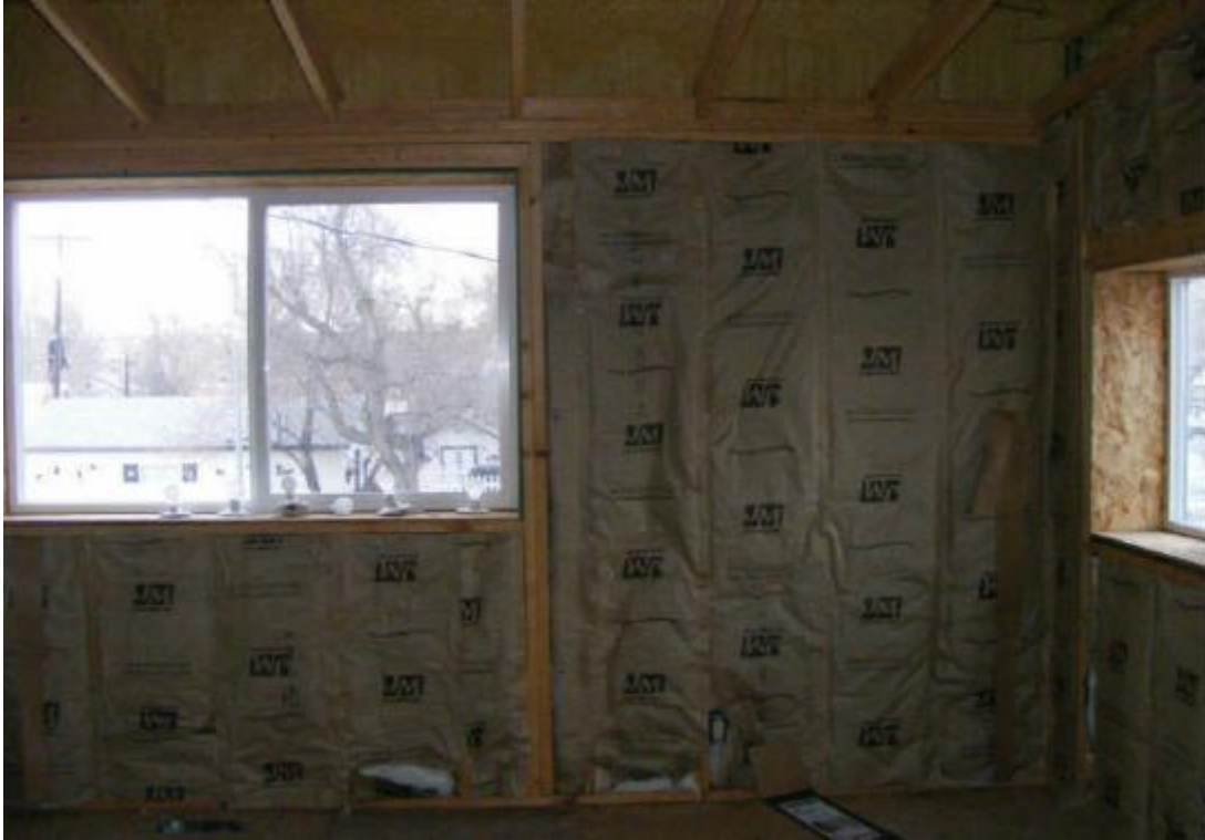
Home – Basement – Unfinished Area
