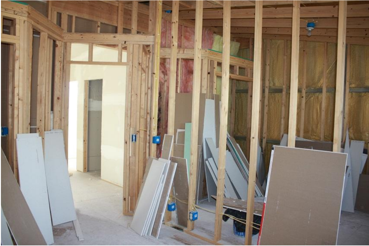
Garage Interior – Upper Level
