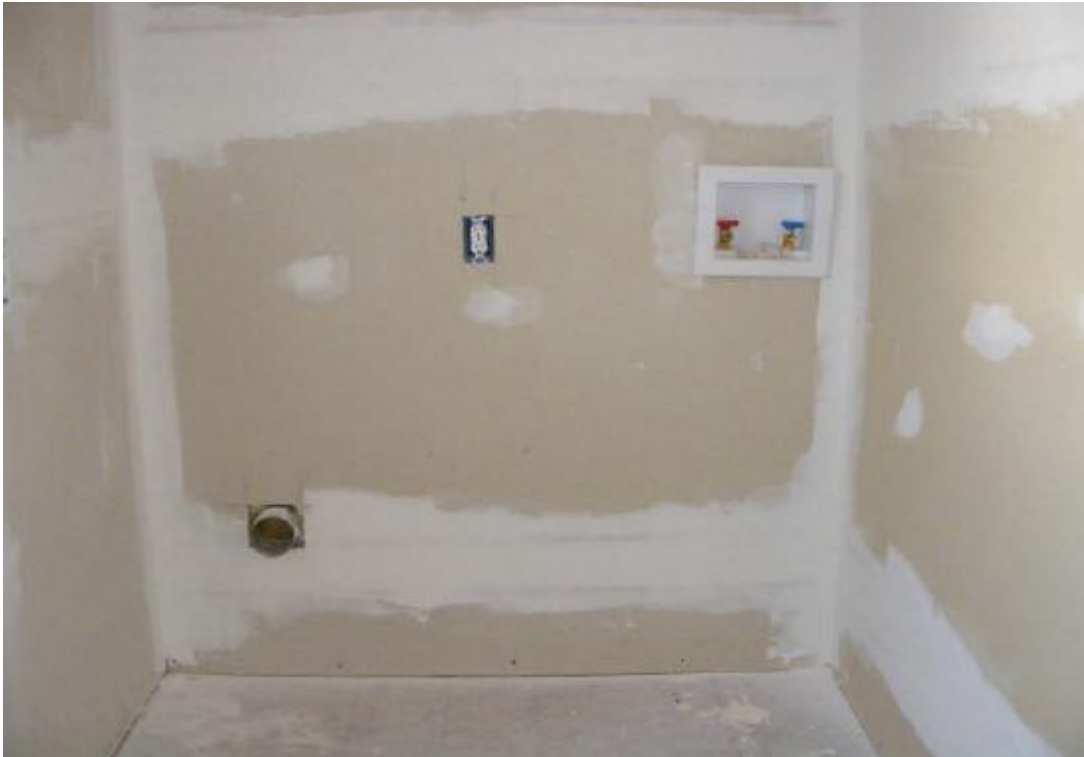
Garage Interior – Upper Level – Unfinished Laundry Room
