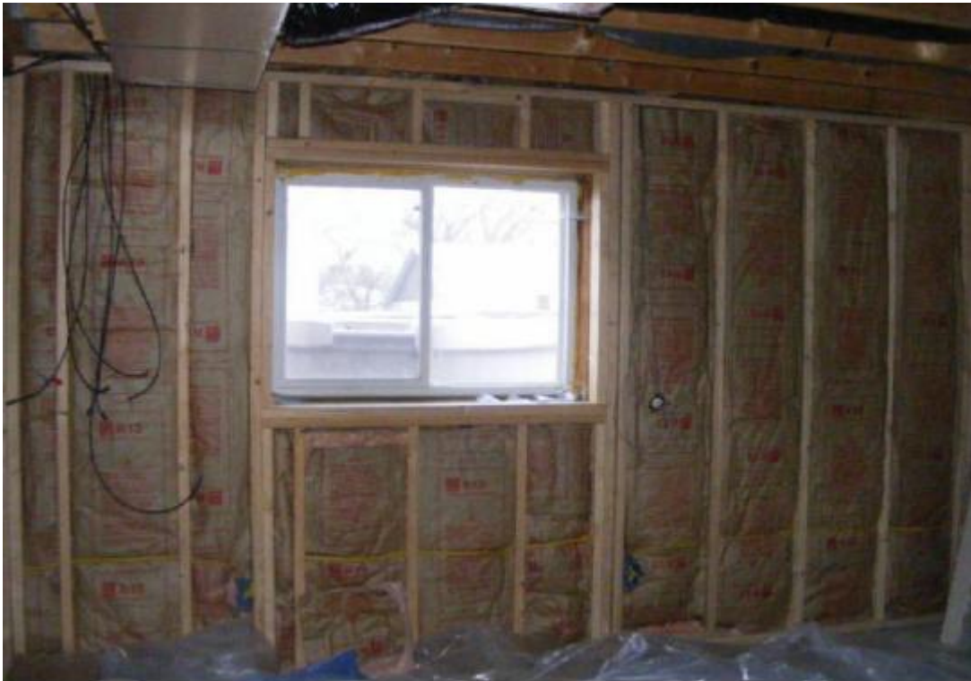
Home – Basement – Unfinished Area
