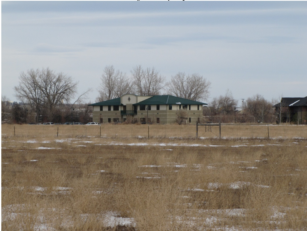
View north and east – Stillwater Mining Corporate office – Transtech Subdivision
