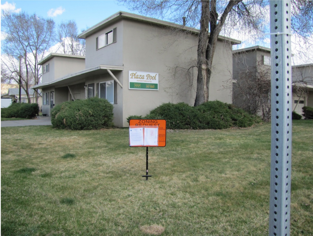
Subject Property – southwest corner at 17 th St W and Avenue E
