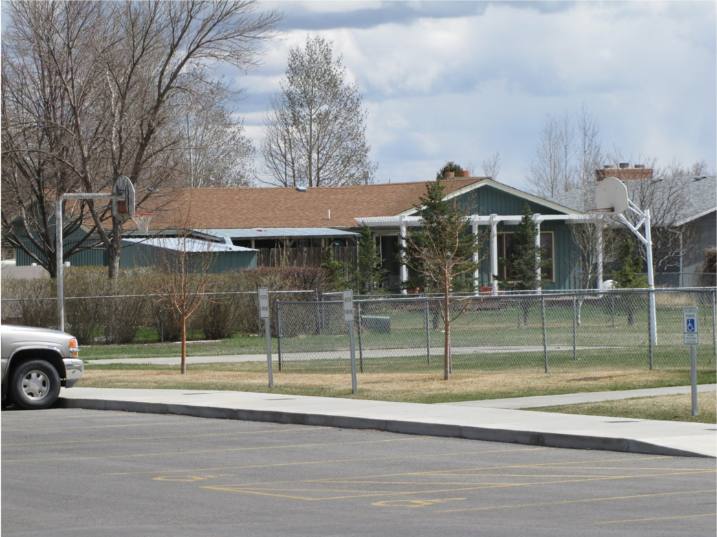
View of east property line – location of future parking lot
