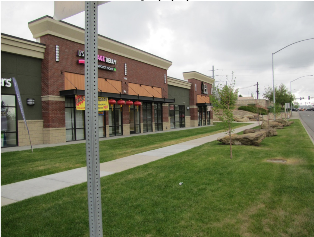
View north along S 24 th St West
