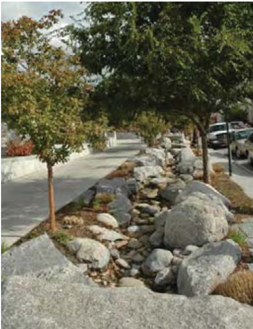
FIGURE 2-3 LANDSCAPED SWALE FOR SURFACE RUNOFF
