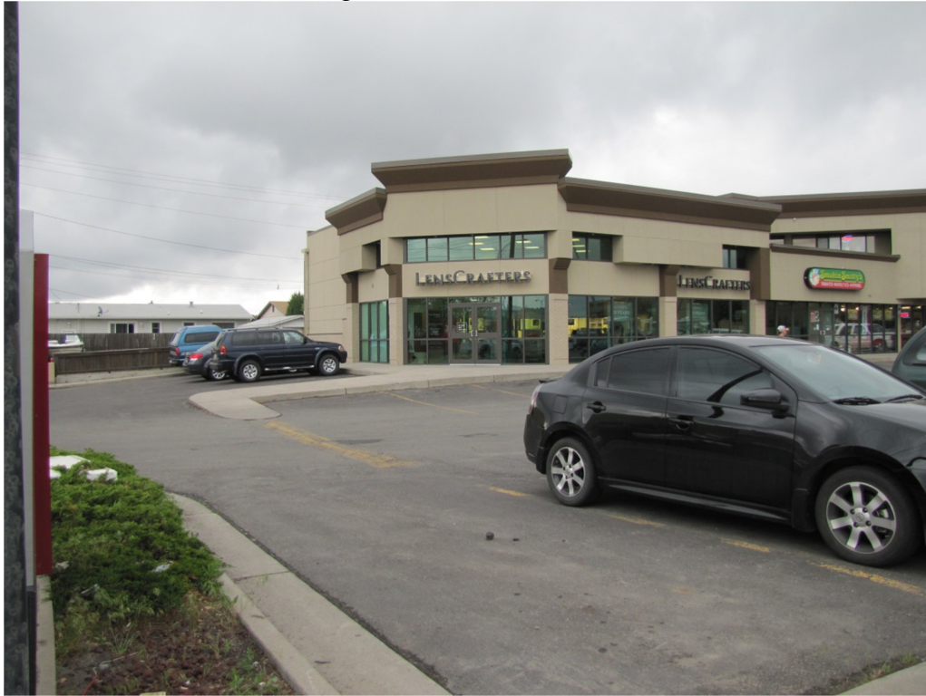
View of north end of existing building
