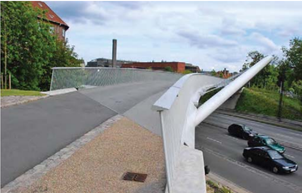
FIGURE 2-20 EXAMPLE OF PEDESTRIAN OVER CROSSING
