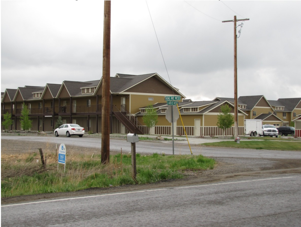
View north and east across King Ave West
