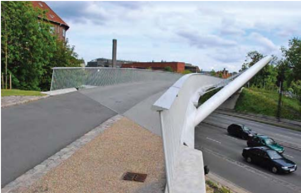
FIGURE 2-20 EXAMPLE OF PEDESTRIAN OVER CROSSING
