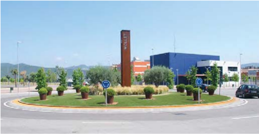
FIGURE 2-27 SPECIAL SIGNAGE WITHIN A ROUNDABOUT
