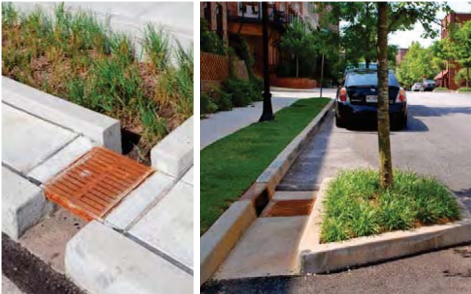
FIGURE 3-2 EXAMPLES OF STORM DRAINAGE IMPROVEMENTS
