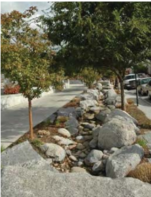
FIGURE 2-3 LANDSCAPED SWALE FOR SURFACE RUNOFF
