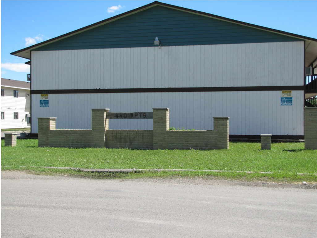
View south across Josephine Drive
