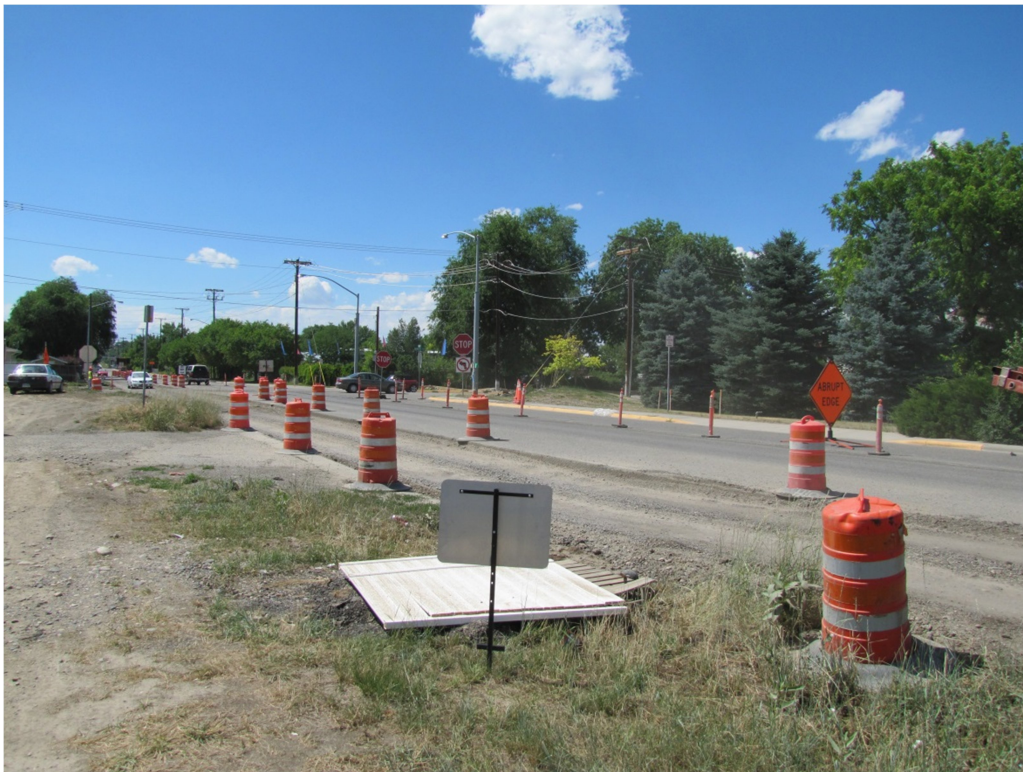
View west along Yellowstone River Road
