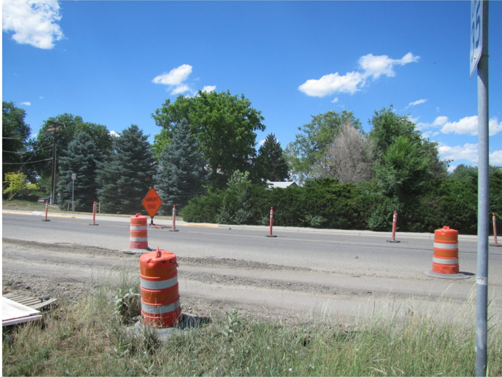
View north across Yellowstone River Road
