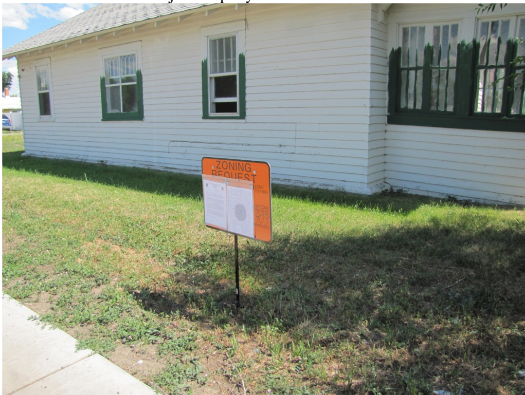
Subject Property – view from State Avenue
