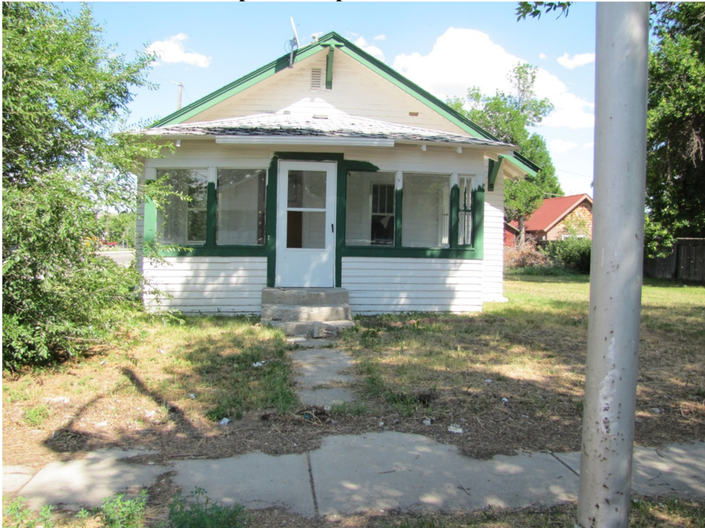
Subject Property – 3 Jefferson Street
