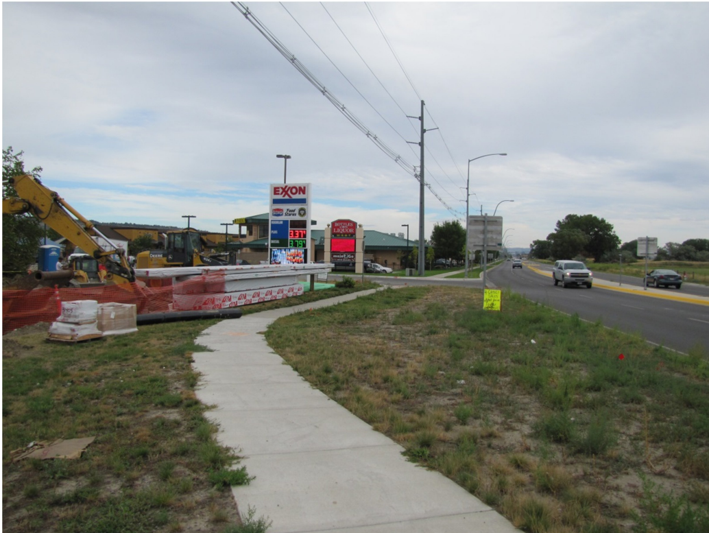
View east along Grand
