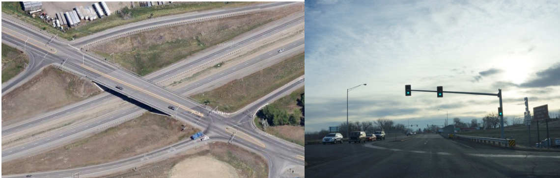
Aerial View (Google Images, 2013); on the ground view of the interchange.
