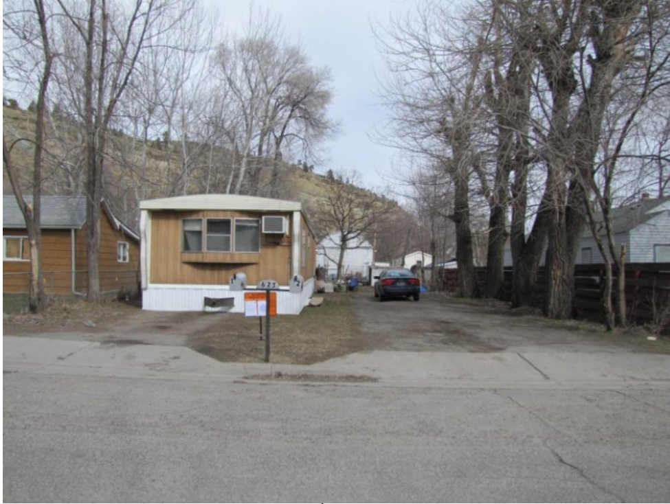
View east across N 15 th Street to subject property
