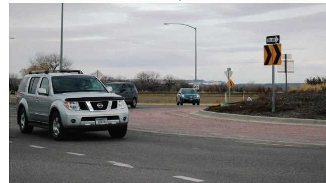
Exhibit 11.12 Roundabout at Airport Road and 27th Street
