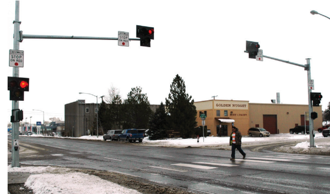
Exhibit 11.11 Pedestrian Hybrid Beacon on 4th Avenue
