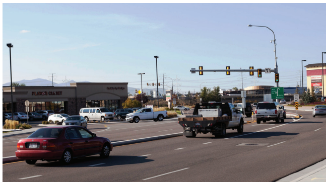
Exhibit 11.9 Median U-Turn intersection in Draper, Utah
