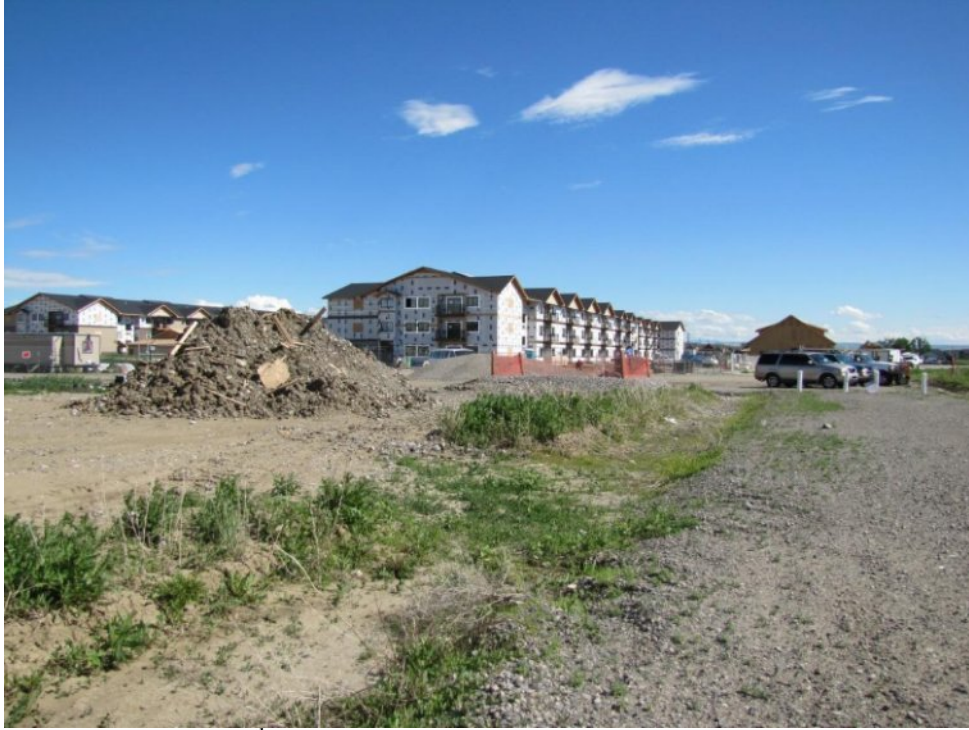
View south along S 44 th Street West – multi-family apartments under construction
