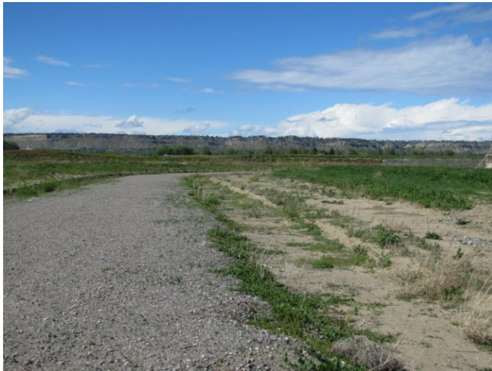
View north along S 44 th Street West – connection to Monad Road
