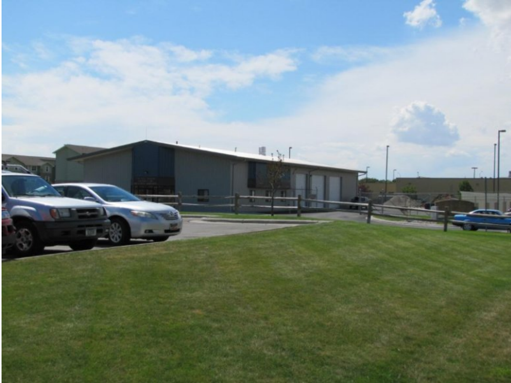
View south and west – Billings Heights Water District offices
